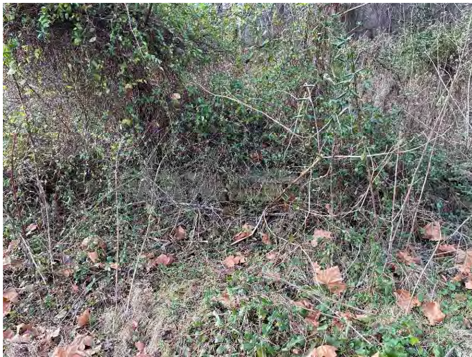
Figure 47: Concrete slab wall built along the trolley bed hill by Francis Smith, partially obscured by brush.
