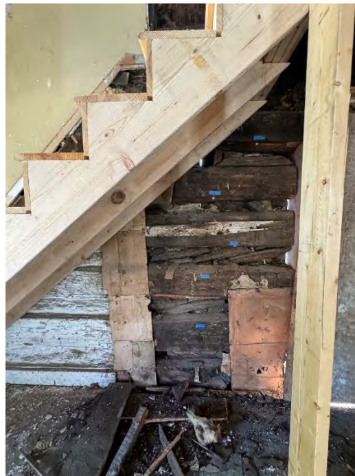
Figure 89: View of the spandrel space beneath the staircase, showing more of the new wood making up the rebuilt staircase. Part of the original horizontal log siding can also be seen through the spandrel. (10 September 2024). Image courtesy of Elizabeth Comer.
