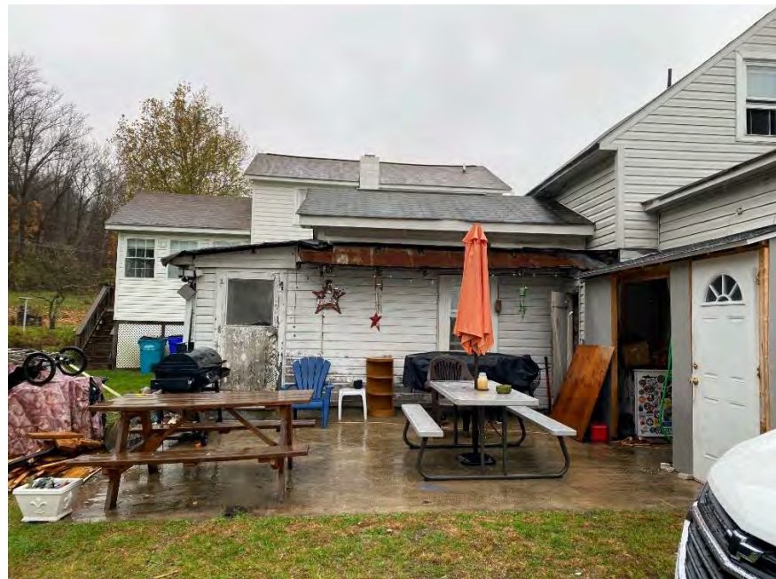
Figure 35: South Elevation of the west addition and the rear patio. The summer kitchen's south window, gable frame asphalt shingle roof, and metal overhang with wooden pole rafters are all visible, as is the anteroom's lean-to roof and screen door. To the right is the lean-to structure covering the crawl space entrance, including both its door and its uncovered opening. (February 2023). Image courtesy of Elizabeth Comer.
