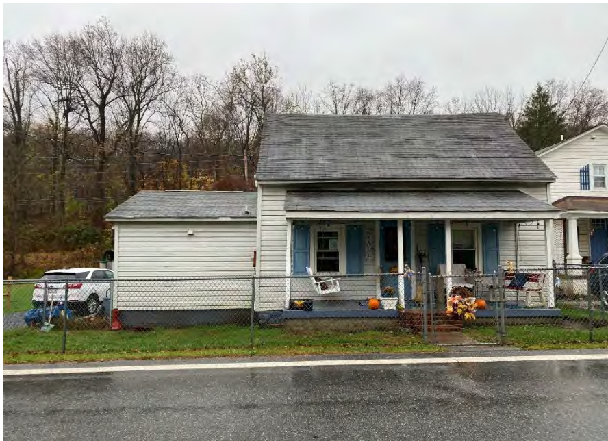
Figure 7: East elevation of the Hoke dwelling, providing a view of the asphalt shingle roof and white vinyl siding, as well as the front porch, door, and windows. Also in view are the south addition, the walkway and steps leading from the road to the front porch, the fence that once surrounded the front yard, and the driveway. The Rohwein infill dwelling is next door on the right. (ca. 2023). Image courtesy of Elizabeth Comer.
