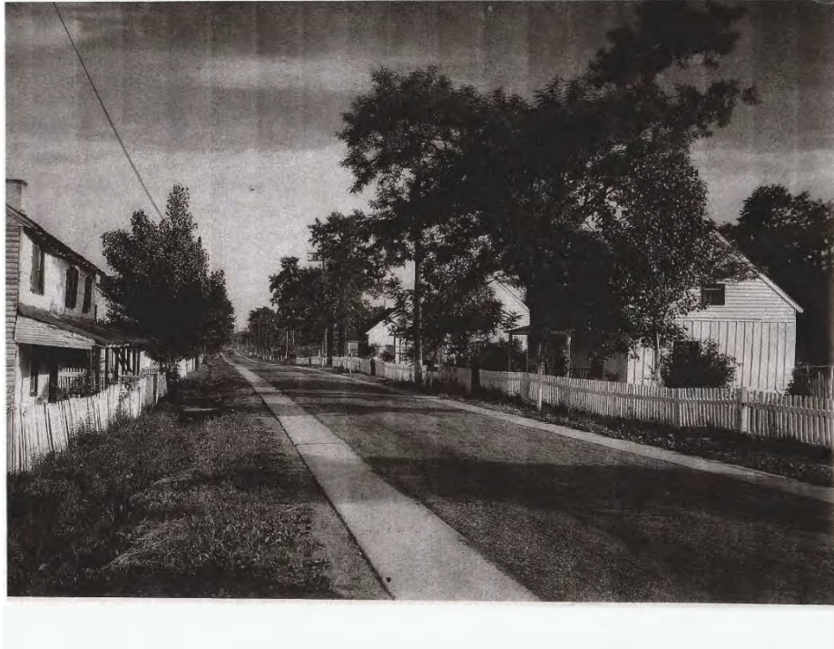
Figure 60: Photograph of Catoctin Furnace Road facing south. While the Hoke dwelling is not clearly visible, note the vertical board and batten siding on the Carty-Miller dwelling (right), which was the original siding configuration. The fence spanning across the front yard is also the earlier, white-painted wood picket fence that existed in front of most of the village houses at the time. (October 30, 1932).
