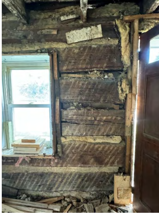
Figure 86: East elevation interior wall between the northernmost front window and the front door post-excavation. Small planks and blocks of wood can be seen intermittently attached to the original log wall. The chinking around the third highest log appears to have deteriorated or otherwise been stripped away, leaving gaps between the logs above and below it. (10 September 2024). Image courtesy of Elizabeth Comer.
