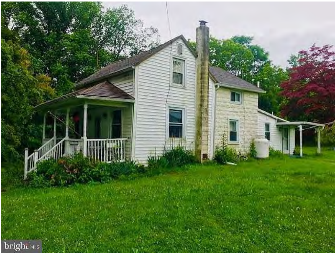
Figure 1: 13204 Catoctin Furnace Road at the southern edge of Mine Bank, built ca. 1900.
