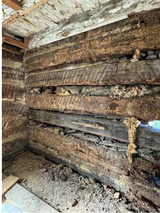
Figure 82: Wider view of the northwest portion of the original structure, showing more of the floor as well as the horizontal log walls, chinking, and some of the hole in the wall where the gas heating system was installed by the Smith family. (10 September 2024). Image courtesy of Elizabeth Comer.
