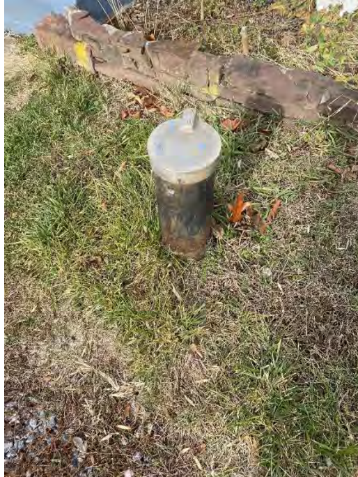
Figure 50: Black well casing between the driveway and south addition.
