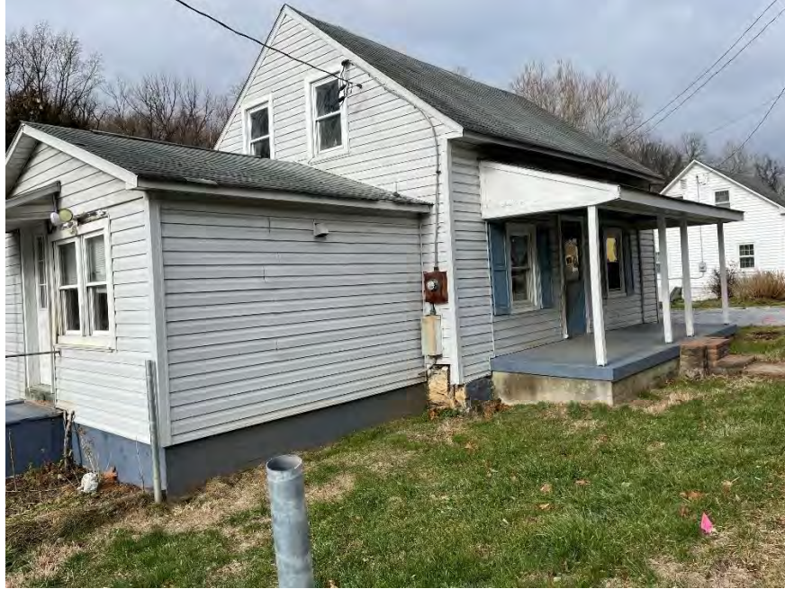
Figure 8: East and south elevations of the Hoke dwelling, providing a closer view of the vinyl siding, the gable frame roof, the front porch, and the porch's lean-to style covering. The two second-story windows on the south elevation can also be seen above the south addition, and two of the former fence posts can be seen in the bottom foreground and at the corner of the south addition.
