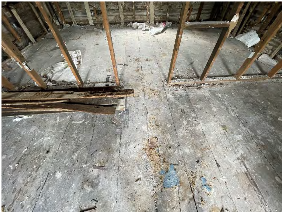
Figure 33: The original upstairs wood floor post-excavation. (25 April 2024).
