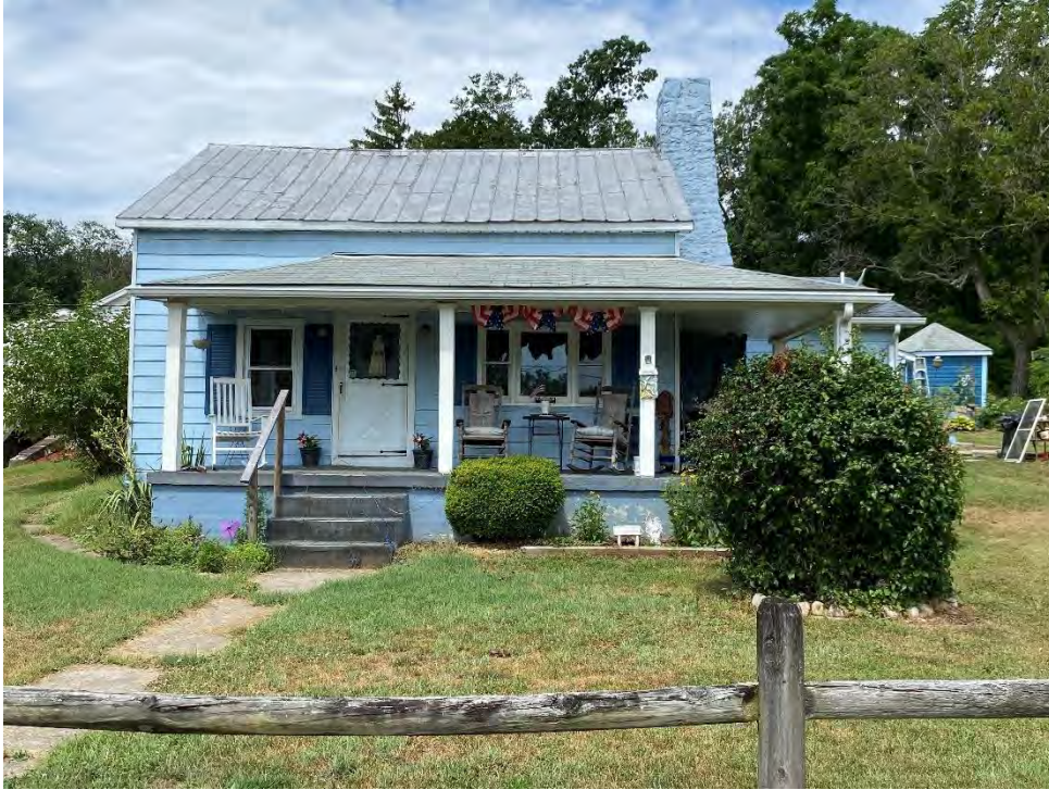
Figure 4: 13230 Catoctin Furnace Road in Mine Bank. Another early 19 th century worker home, its original historic hearth and chimney are still fully intact on the right. Image courtesy of Elizabeth Comer.
