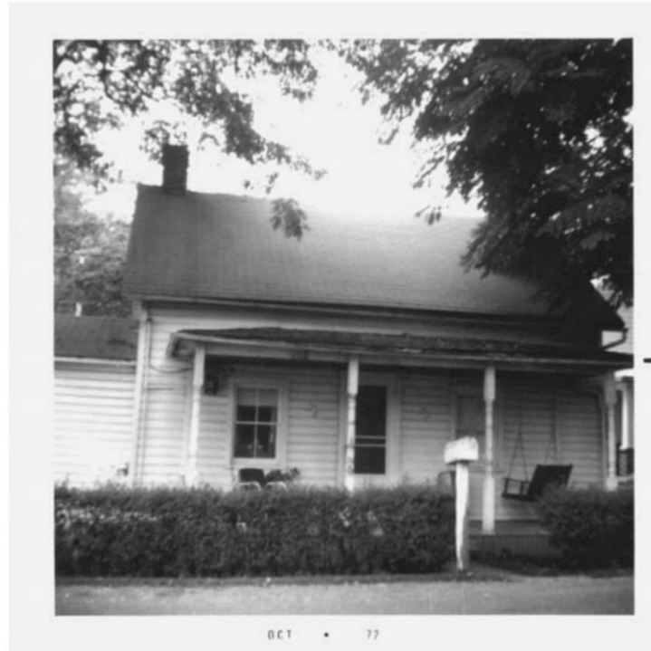
Figure 64: East elevation of the Hoke dwelling, with its earlier all-wood front porch, boxwood shrub front yard hedges, and top portion of the original stone chimney stack all still present, although the chimney was not connected to a fireplace by that time. (October 1972). Image courtesy of Catocctin Furnace Historical Society, Inc.
