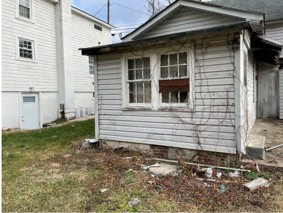
Figure 36: West elevation of the anteroom, showing its double window, white vinyl siding, and brick foundation. In the background to the right is the metal overhang as well as the outside tool closet.
