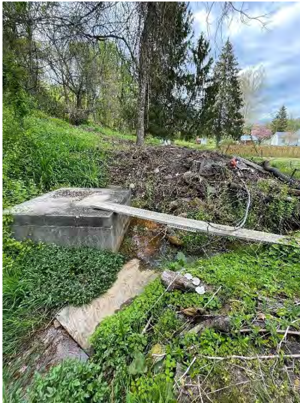
Figure 59: Concrete intake structure just outside the Hoke and Sweeney properties, showing the channel surrounding and flowing south from it. (25 April 2024).
