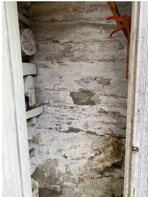
Figure 13: Inside the outdoor tool closet, revealing part of the dwelling's original log construction. (19 December 2023). Photograph by Elizabeth Comer.
