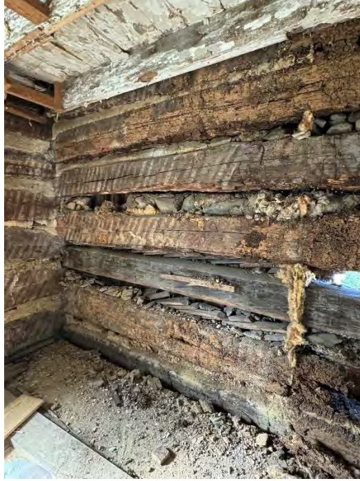
Figure 82: Wider view of the northwest portion of the original structure, showing more of the floor as well as the horizontal log walls, chinking, and some of the hole in the wall where the gas heating system was installed by the Smith family. (10 September 2024). Image courtesy of Elizabeth Comer.
