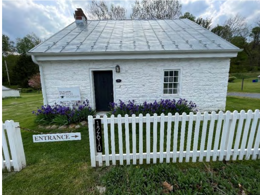
Figure 66: The Museum of the Ironworker at 12610 Catoctin Furnace Road, another historic worker home in the village that shows the original placement of the front door, as well as the original hand-crimped standing seam tin roof. (25 April 2024).
