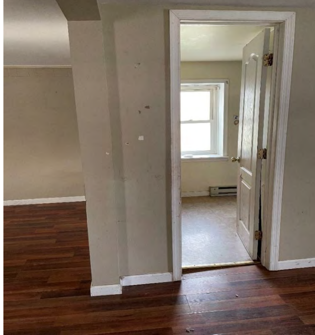
Figure 16: The entrance to the restroom, displaying its single window and linoleum tile floor. The southern portion of the boxed header can also be seen left of the restroom door.
