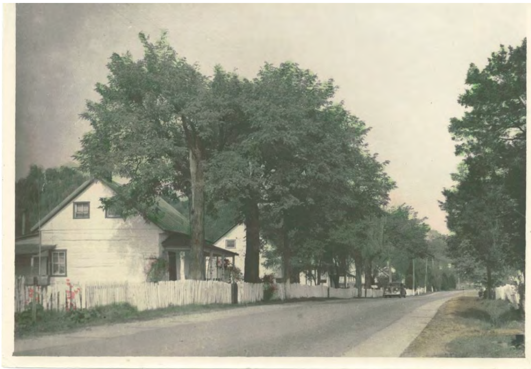
Figure 63: Hand-colored photograph of Catoctin Furnace Road facing north. The Hoke house is in the left foreground, and can be seen with its small frame shed roof west addition and without its south addition. The earlier front porch installed by Phil Miller, the white-painted wood picket fence, and two large trees that were in the front yard are also visible. Furthermore, the original placement of the front door is present in this image (October 30, 1932).
