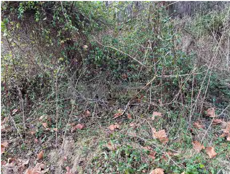
Figure 47: Concrete slab wall built along the trolley bed hill by Francis Smith, partially obscured by brush.
