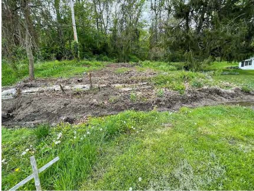
Figure 58: Trolley bed hill in the Hoke rear yard post-excitation. The concrete slab wall, waterflow from the rusted grate, disarticulated culvert pipes, and then extant cross are all visible. (25 April 2024).
