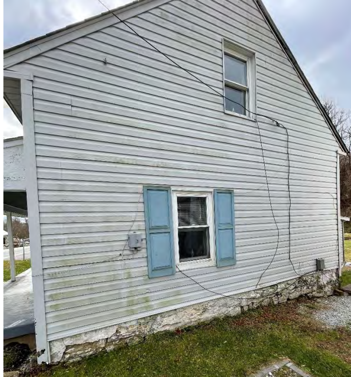
Figure 10: North elevation of the Hoke dwelling, showing the different positioning of the first- and second-story windows, as well as a portion of the dwelling's original stone foundation.
