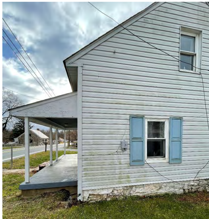
Figure 9: North elevation of the Hoke dwelling, showing the first- and second-story north elevation windows, and providing a profile view of the front porch.
