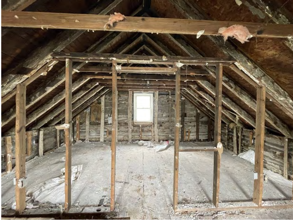
Figure 32: Upstairs wall and doorframe post-excavation, facing north. (25 April 2024).
