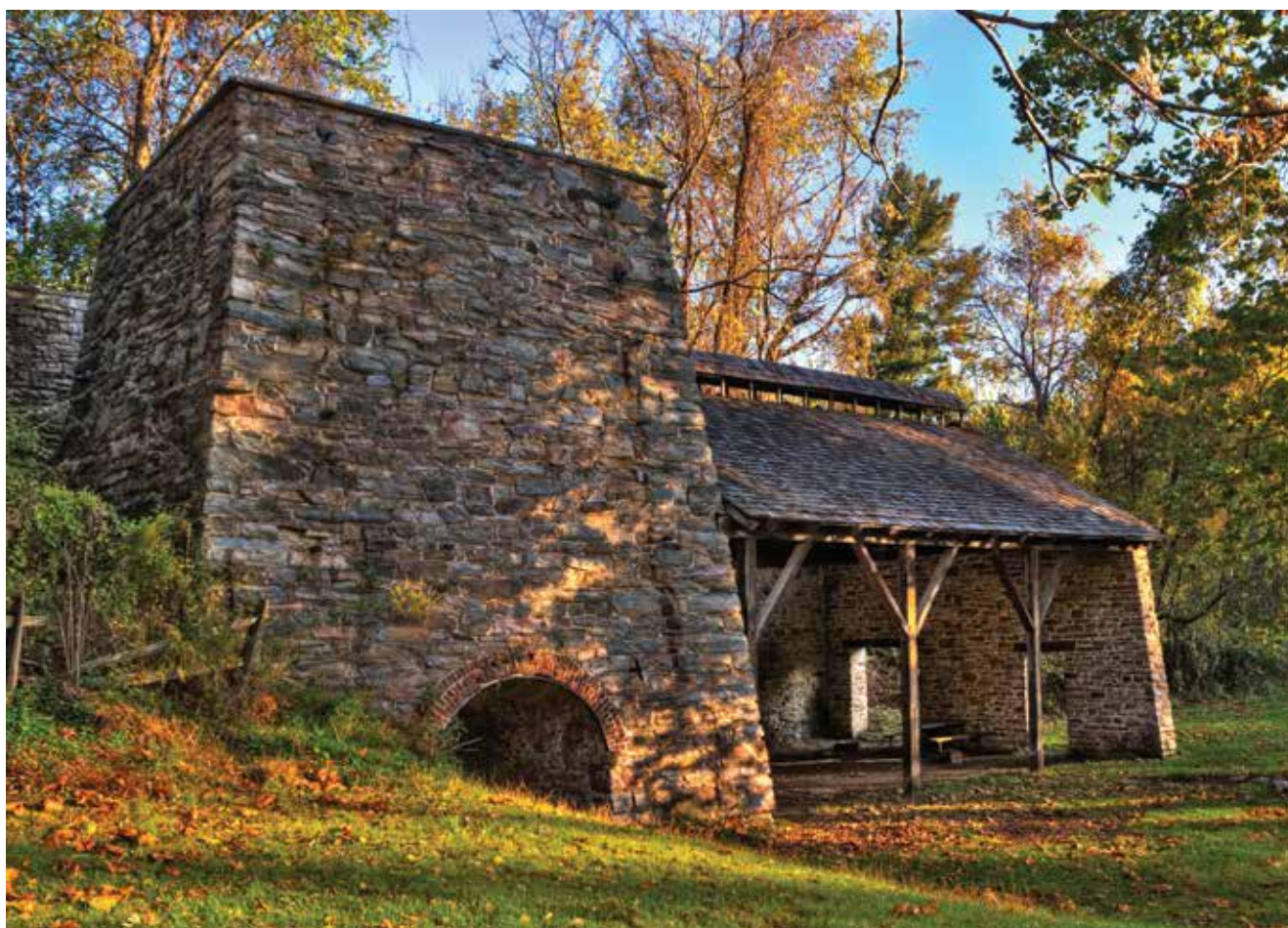
A 33-foot-high furnace stack named Isabella, next to its reconstructed casting shed, was originally built in 1857 and remained in continuous blast until 1893.
