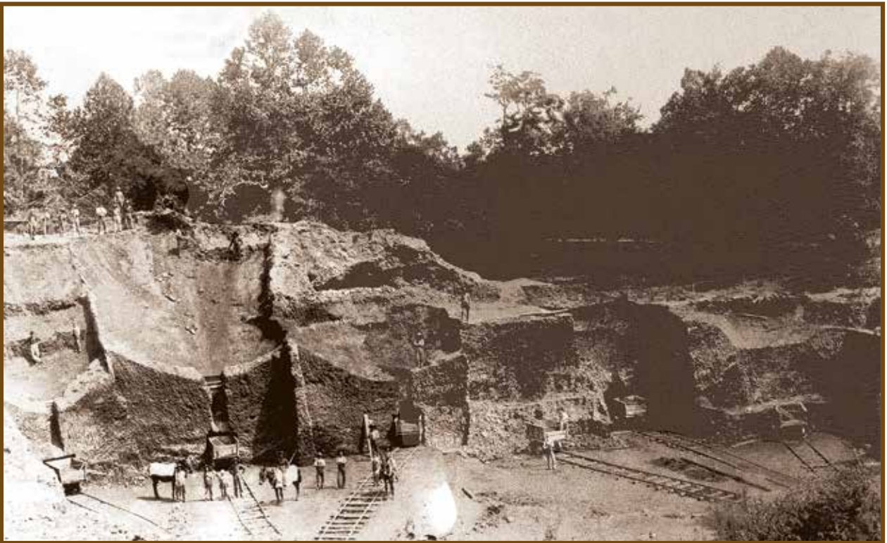
Iron ore for Catoctin Furnace was mined from three ore banks using mule-drawn carts. This ore pit reached a size of 500 by 200 feet with a depth of 20 feet. Recent research has allowed more accurate artifact dating by tracing zinc and other minerals to specific ore banks.
