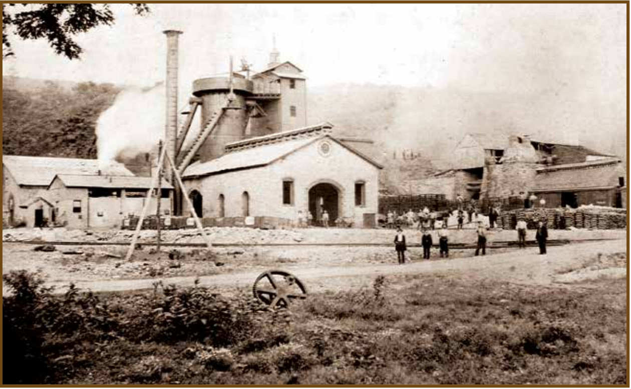
Catoctin Furnace, circa 1890, shows a vibrant operation with furnace stack, Deborah, left, in blast. Pig iron sits in stacks near the Isabella furnace, right, which still retains its boiler and air heater, but is not in operation.
