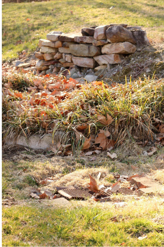
Figure 38: The grate's position in regard to the paper burn pit.
