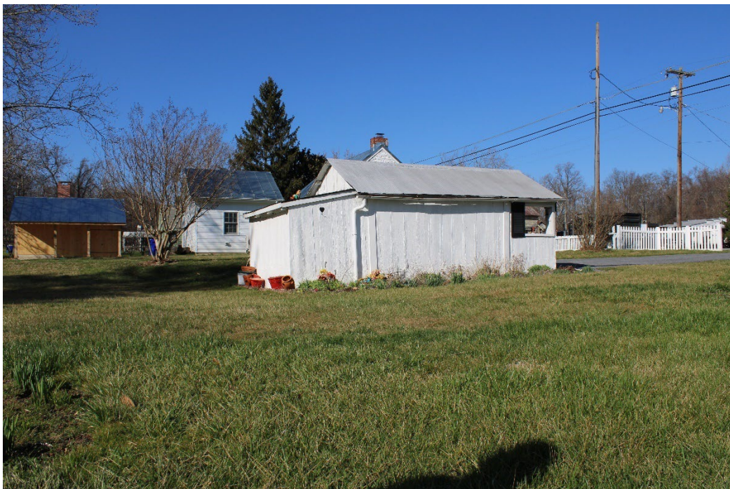
Figure 9: Photograph of the garage, facing northeast. The main gable-framed roof and rear lean-to style roof are both visible, as are the flowers and shrubs planted along its south side, the pots stacked on its west side, its window opening, and the crawling gnome. To the right, the driveway and the driveway opening in the fence can be seen. In the bottom left corner is the outline of the old flower bed.
