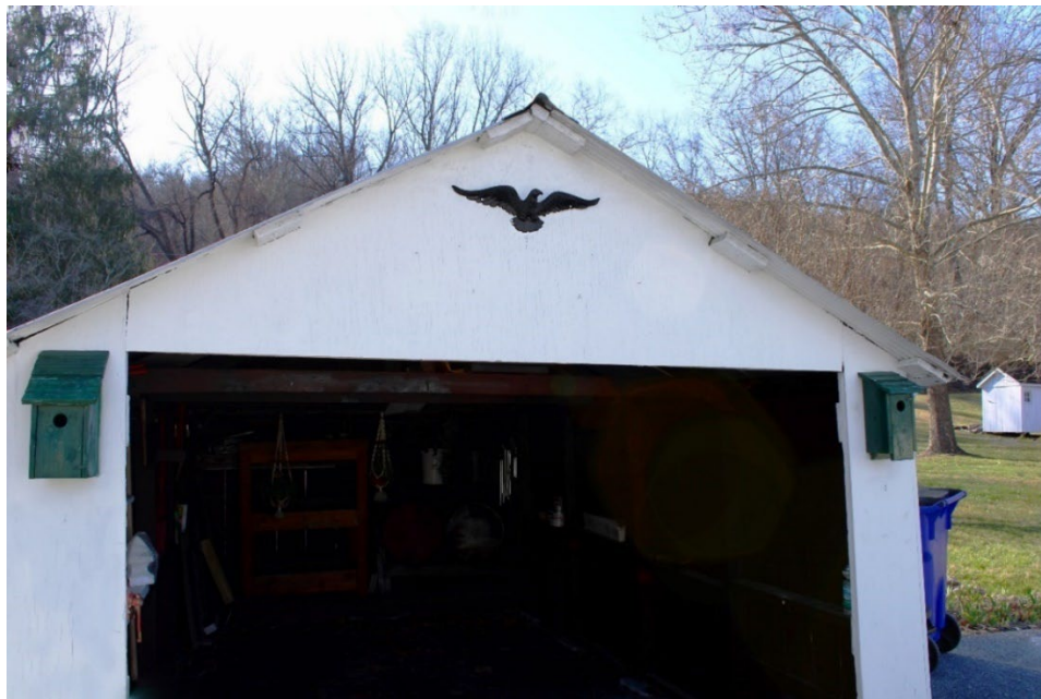
Figure 11: Front view of the garage, showing its short "door" opening, gable-framed roof, the two bluebird houses on either side, the metal cast eagle hanging over it, and some of the flowers planted at the end of the driveway to the right. The inside is also slightly visible, though heavily shaded.
