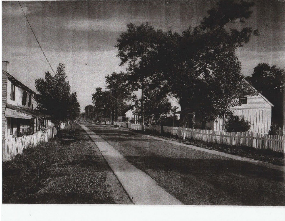
Figure 52: Photograph facing south, showing Carty-Miller house on right side. Note the vertical board and batten siding, and original window placement are all still present on the house. The fence spanning across the front yard is also the earlier, white-painted wood picket construction. (October 30, 1932).
