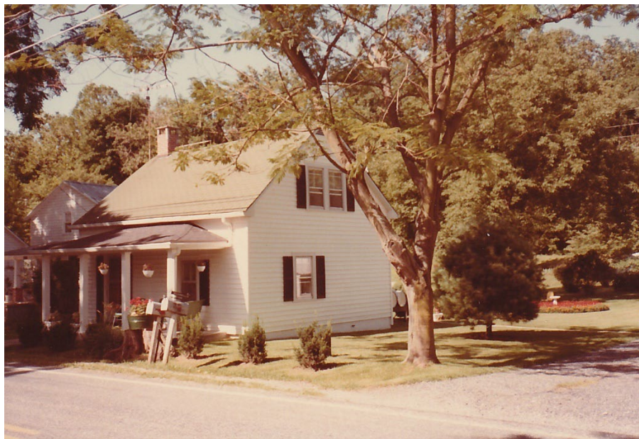
Figure 55: The Carty-Miller front yard, showing several changes made by Clint Miller, such as the front porch, second story double window. The large mimosa tree is in the foreground beside the driveway, with the small pine tree visible behind it. To the left of the two mailboxes is the stump of the locust tree, with a flower pot placed on top of it. Farther in the background, the flower bed and birdbath, as well as the kerosene barrels, can be seen. Photograph taken some time after the vinyl siding and black shutters were added in 1982. Note: Southernmost chimney is still extant near the top left.
