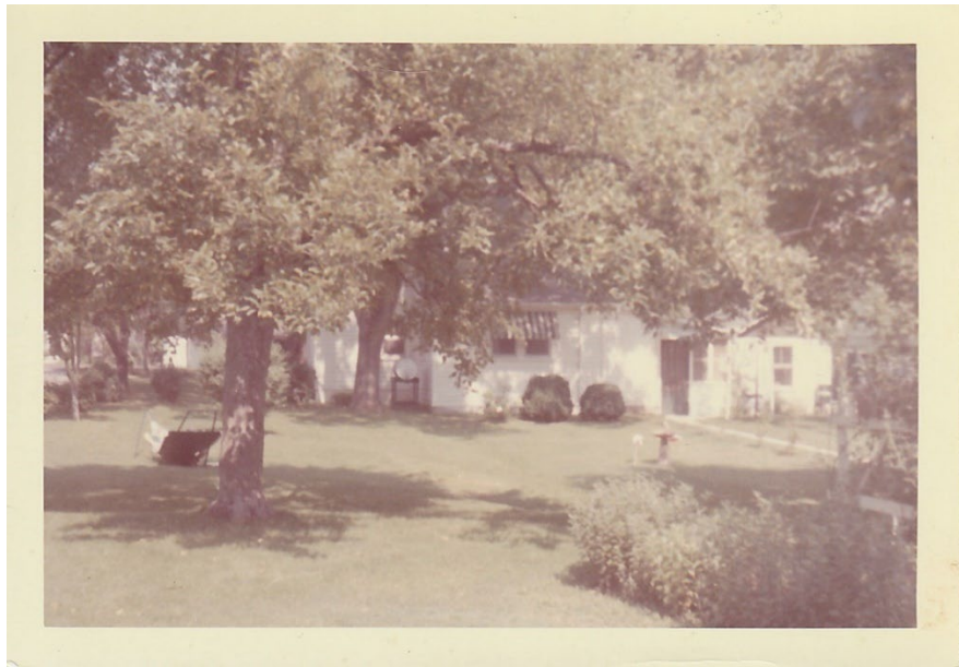
Figure 53: Photograph of the Carty-Miller rear yard and west side of the dwelling. The dwelling's German weatherboard siding can be discerned over the original log siding. The breezeway, with its door held ajar, the "summer kitchen," and the double kitchen window, which were all relatively recent alterations to the dwelling can also be seen. The barrel which fueled the original kerosene heating system can be seen tucked in the corner left of the kitchen window. Also visible are the birdbath before flowers were planted around it, an apple tree (left) and a walnut tree beside the barrel. (July 1963).
