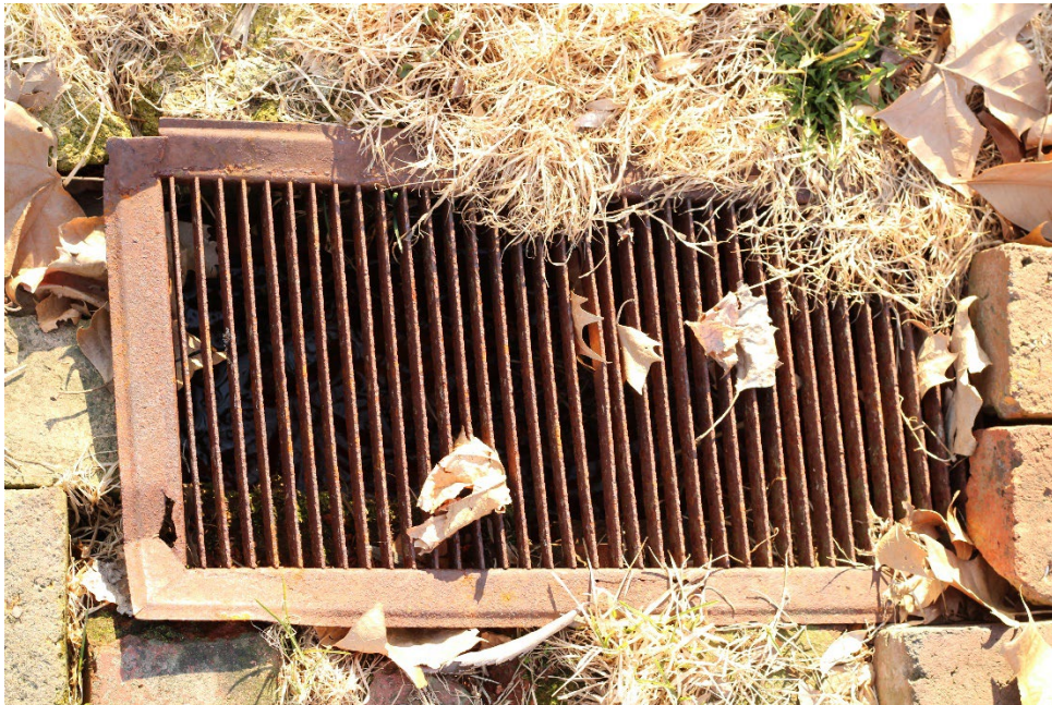
Figure 37: Close-up view of the grate by the paper burn pit. Rainwater can be seen puddling below it.
