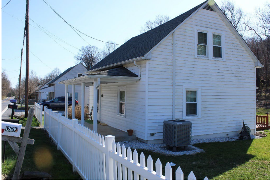
Figure 2: The front of the Carty-Miller dwelling facing south. The covered front porch, the white vinyl picket fence, the white vinyl house siding, the asphalt shingle roof, the second-story double window installed by Clint Miller, the first-story window, and the newer A/C unit are all visible in the foreground. The rear deck is also slightly visible in the far right, while the front door and window can be seen to the left. Also to the right is the spigot connected to a hose that was installed after the Miller family had the well drilled in 1977.
