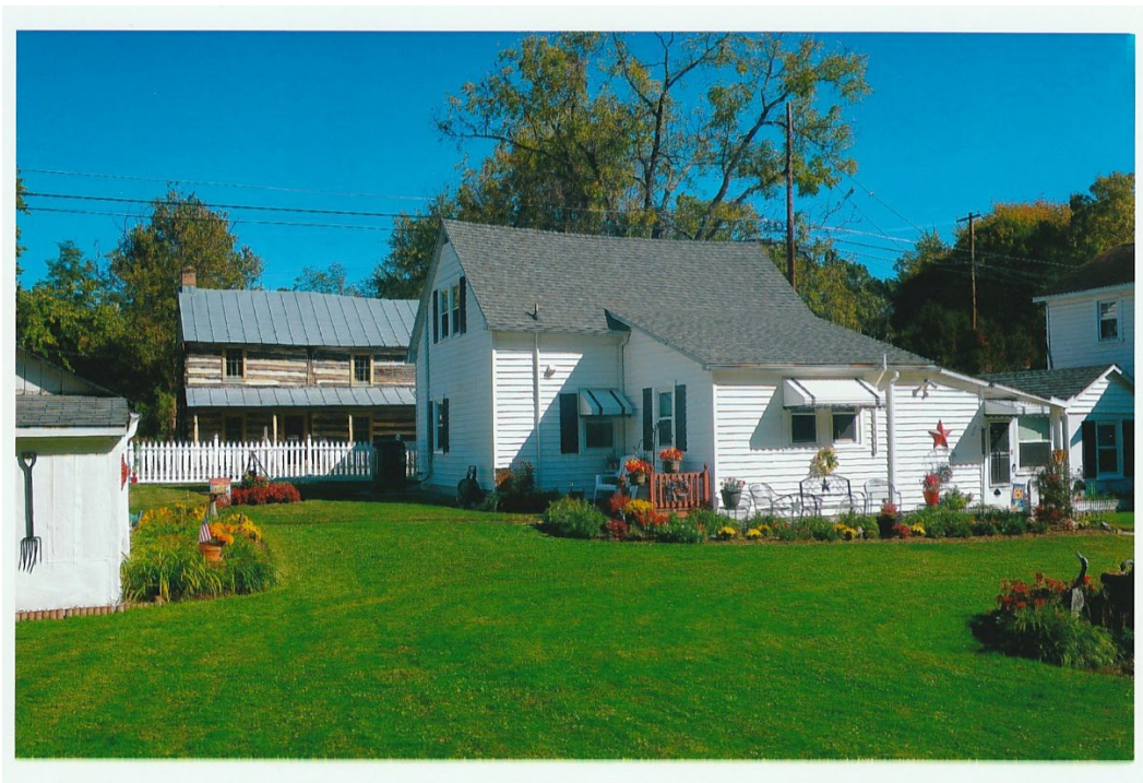
Figure 7: View of the dwelling from the northern rear yard. The awnings on the breezeway door, kitchen window, and window over the back deck are all visible, as are the shutters on the two windows on the north elevation of the dwelling, the two above the back deck, and the one on the laundry room. Chimneys have both been removed above roof line. Various gardens, lawn ornaments, and exterior house decorations can be seen, such as the red star to the left of the breezeway door. (ca. 2021). Photograph by Joann Miller.
