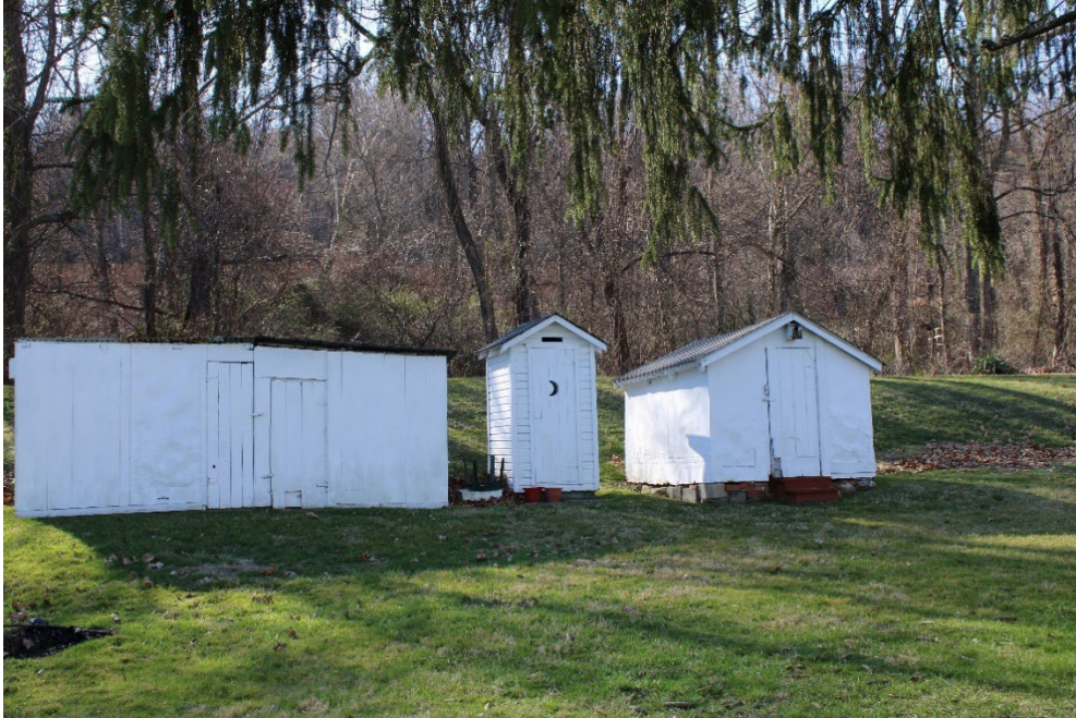
Figure 26: The three outbuildings at the western edge of the rear yard. From left to right: The chicken coop, the outhouse, and the hog pen.
