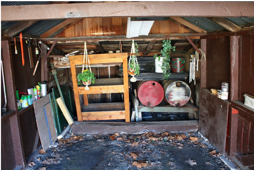
Figure 15: Wide-angle view of the garage interior, showing the railroad tie, potting shelves, two old kerosene barrels, hanging flower pots, and other miscellaneous tools and appliances.
