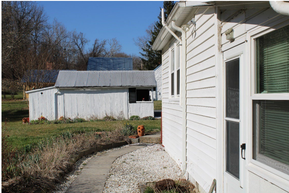
Figure 19: View of the garage from the concrete walkway along the west side of the dwelling, with the gardens on either side of it in the foreground. The breezeway door is also visible immediately to the right, with the double kitchen window a short distance away from it.
