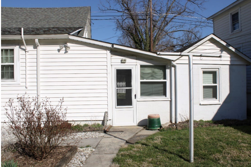
Figure 6: A close-up view of the breezeway and laundry room, facing east from the rear yard. Also in view are the intersection between the two concrete walkways, some of the gardens surrounding the walkway, and the easternmost clothesline pole.
