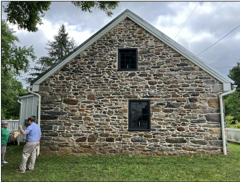
Figure 4: Side wall of the Forgerman's House showing rubble exterior wall.
