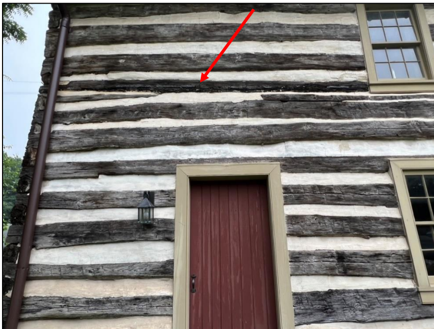
Figure 17: Log that is rotted. See figure below for water that has entered interior from this area.
