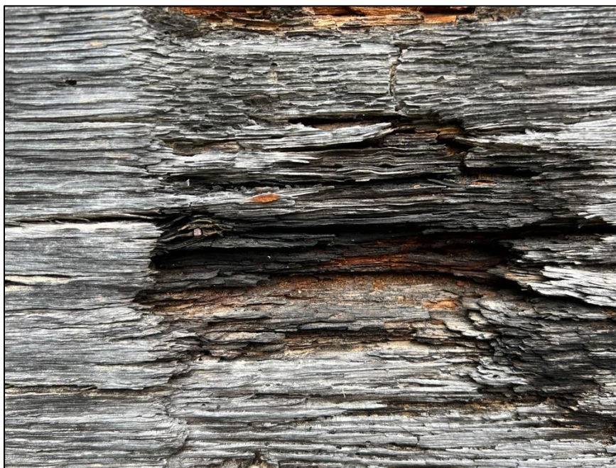
Figure 16: Frass found at area of rot in log.
