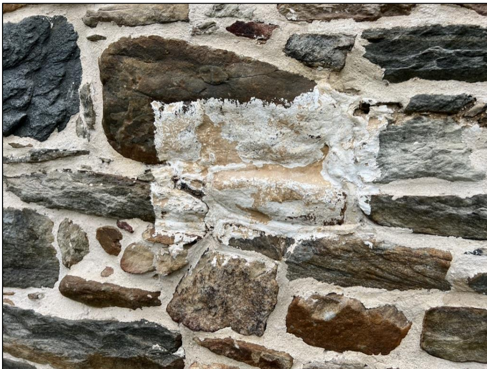
Figure 5: Detail of rubble wall with small section of old limewash or whitewash coating.
