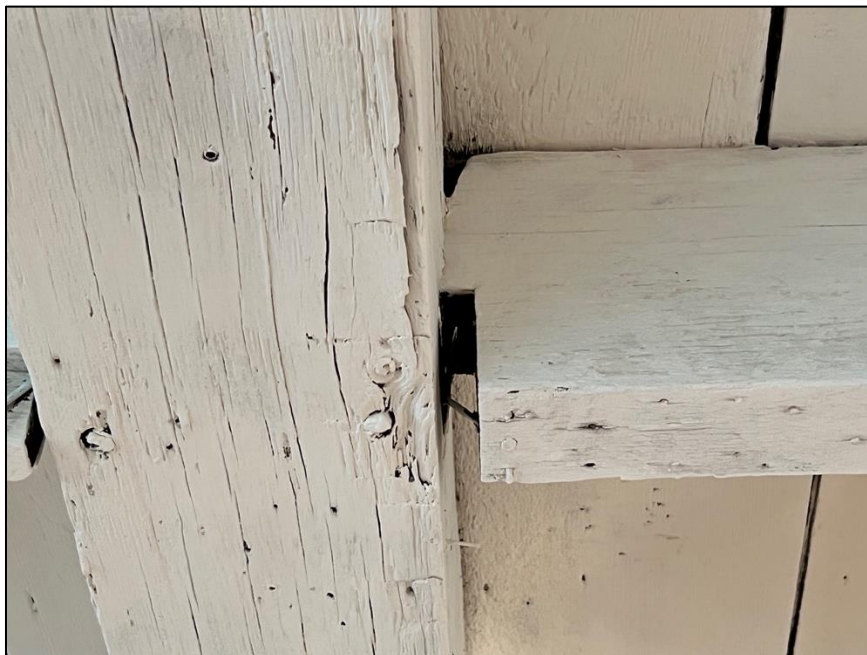
Figure 7: Floor joist with a V bevel tenon. Typical for the second floor joist. Several have pulled away as is shown above.
