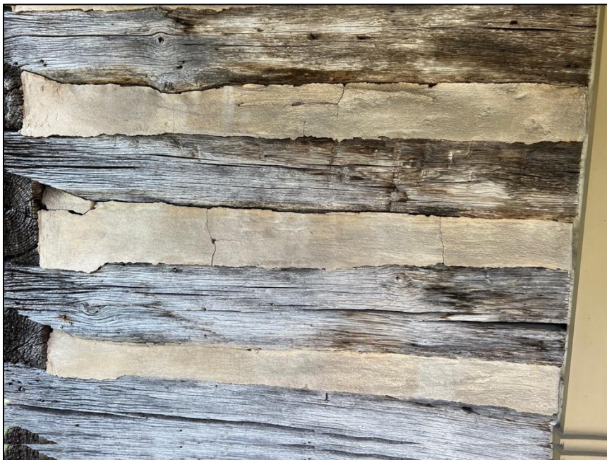
Figure 14: Deteriorated chinking.
