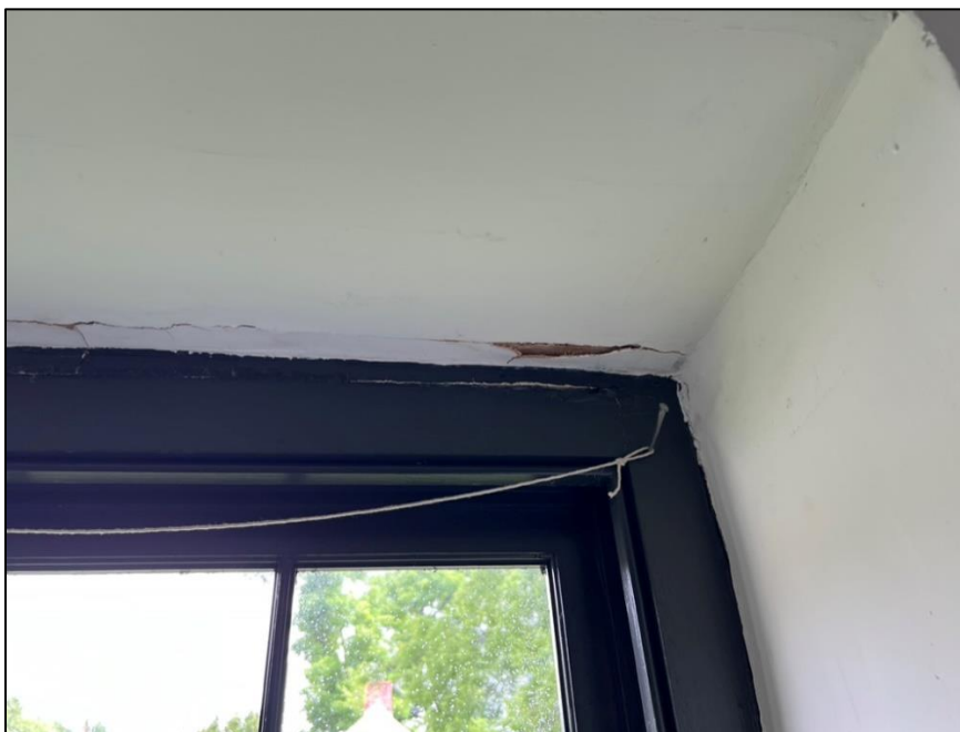
Figure 11: Signs of water infiltration over window.
