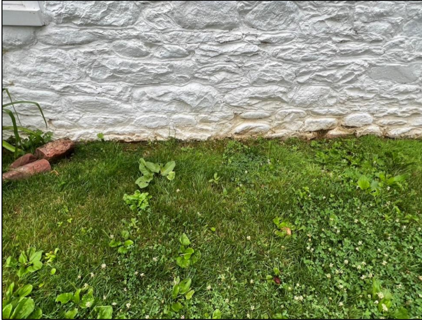
Figure 6: Painted finish beginning to lift at bottom of wall where it meets the soil.
