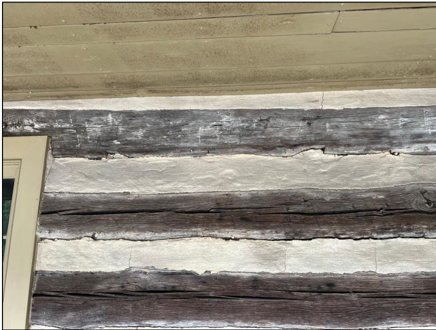
Figure 13: Logs with significant checking.
