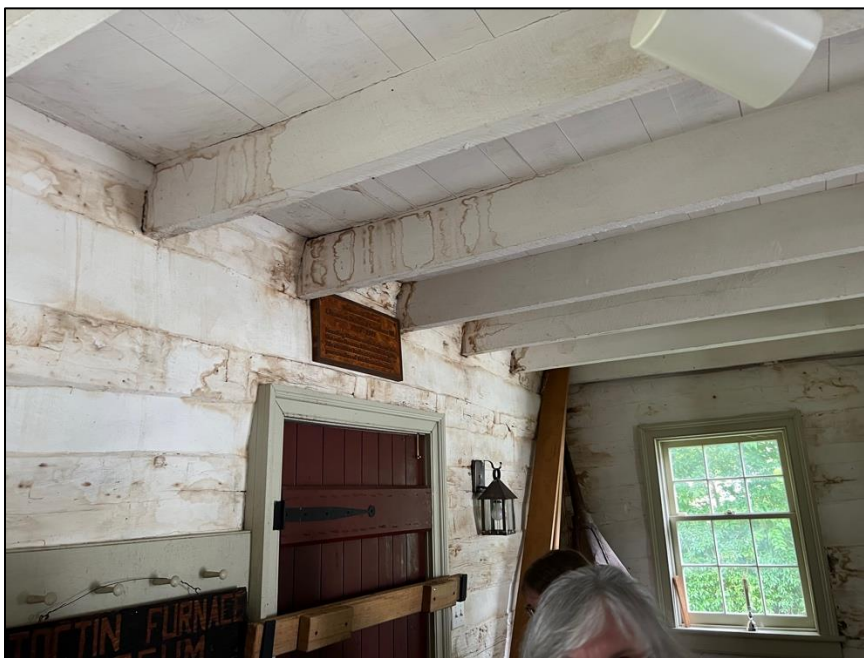
Figure 18: Water staining from water infiltration through rotted exterior logs.
