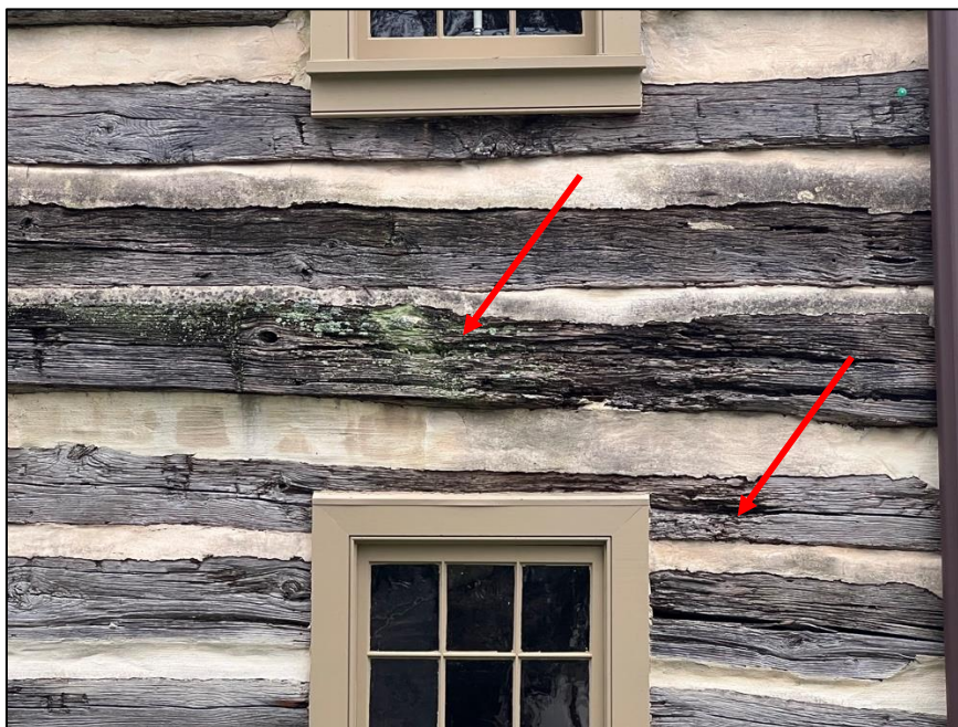
Figure 15: Wood that has rotted and is now hosting biological growth where noted with arrows.
