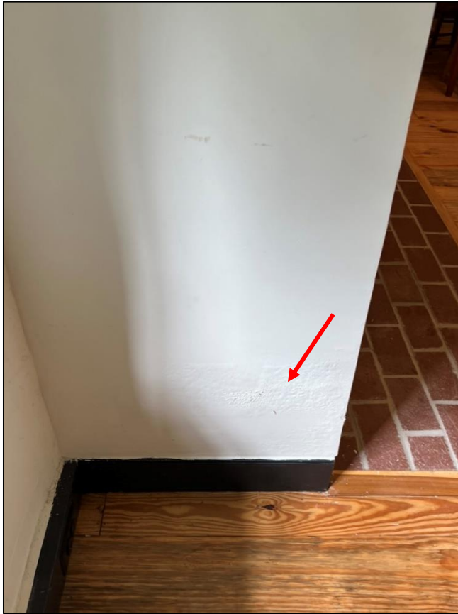
Figure 12: Signs of water infiltration at chimney.
