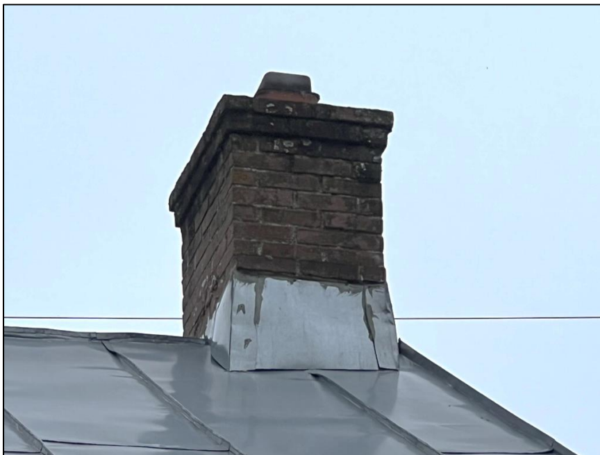
Figure 19: Chimney flashing on Collier's House installed with fasteners and caulk
