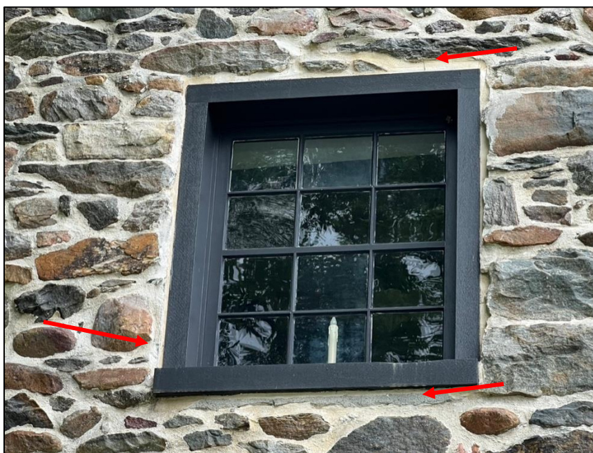
Figure 9: Cracks in mortar over window, mortar repair failing under window, and failure of mortar at side of window.
