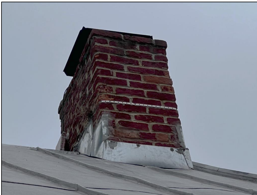
Figure 10: Chimney flashing installed on chimney with fasteners and caulk. Not in the masonry.
