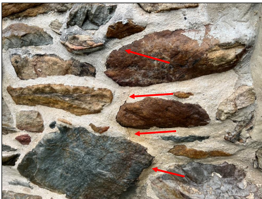
Figure 8: Cracks in the exterior rubble wall mortar. Found in multiple locations.
